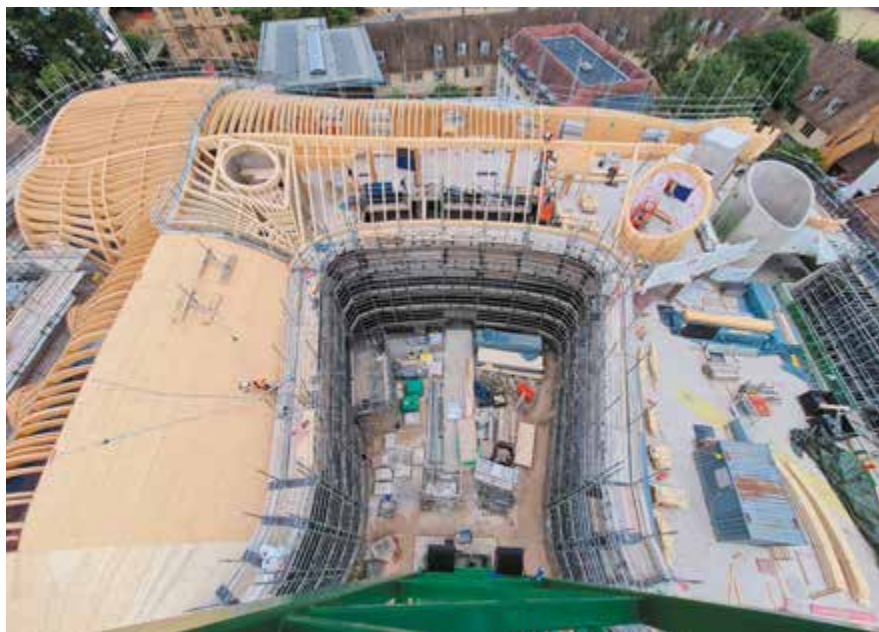
Timber roof of Main Quad under construction
